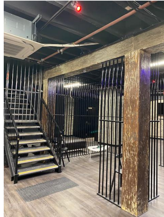
stairs constructed to connect to the tenancy above
