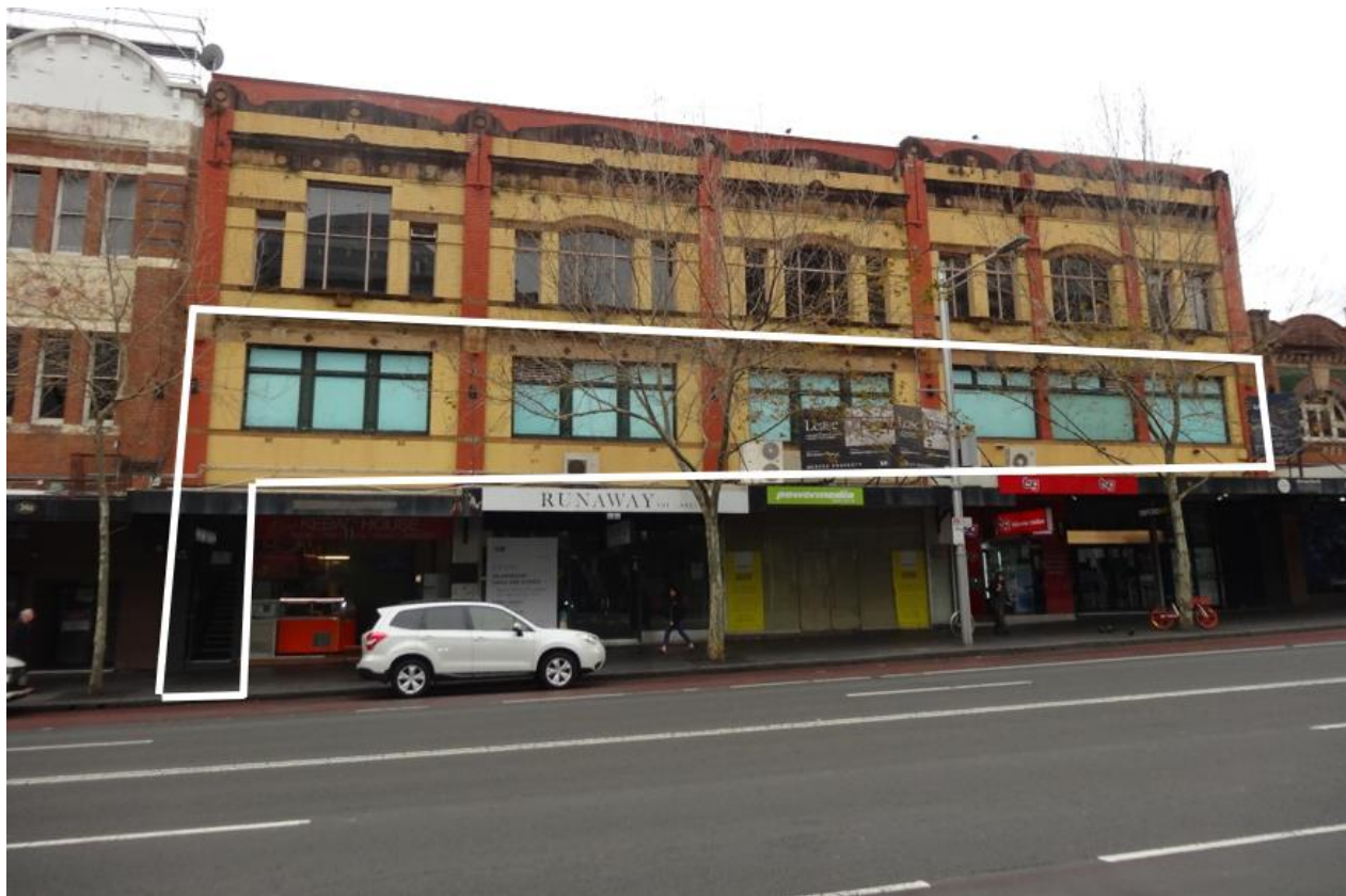
site viewed from Oxford Street
