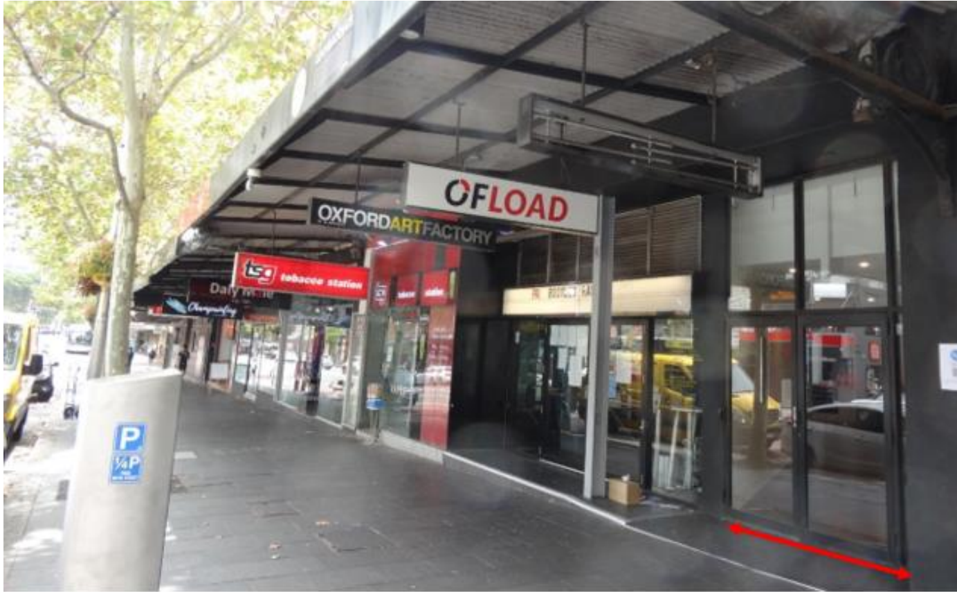
entrance to common corridor and lifts
