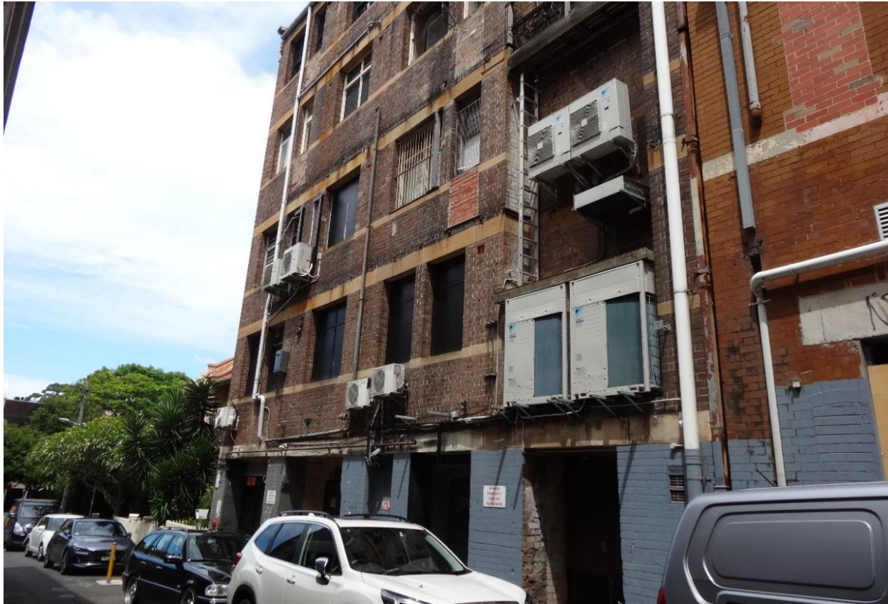
site viewed from Winns Lane
